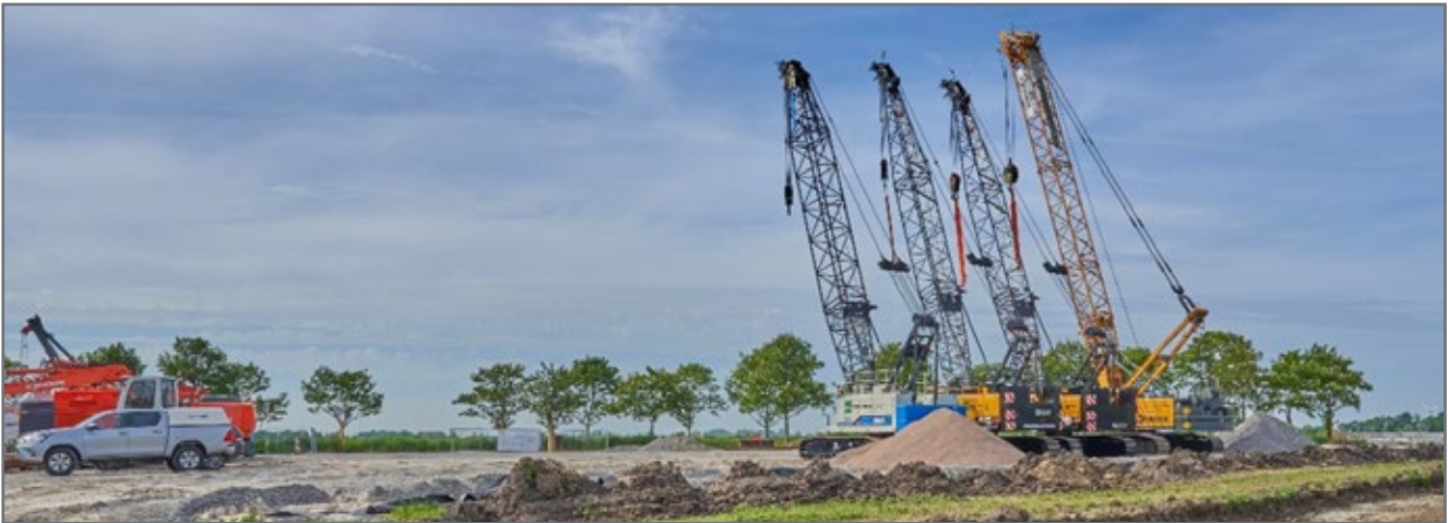
Figure 3: The short construction time required considerable machinery.
