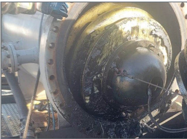
Figure 6: A brush pig being removed
