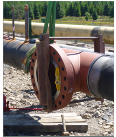
Figure 14: Setting up slit tee for welding at DNV Spadeadam
