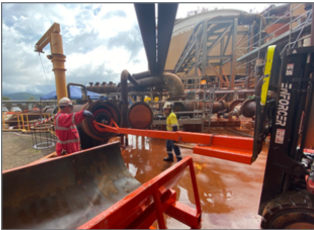
Figure 2: Launcher location during launch of gauging bidi
