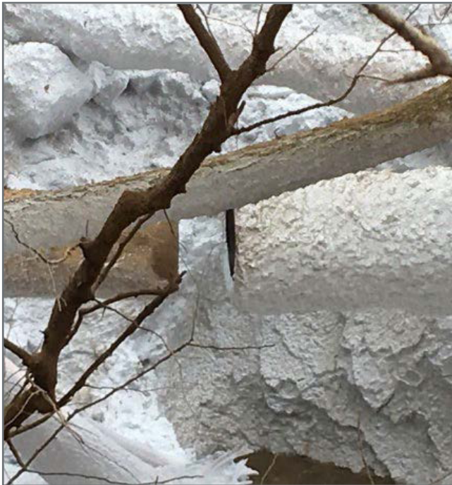
Figure 6: circumferential fatigue crack in a CO2 transport pipeline due to ground movements [6]
