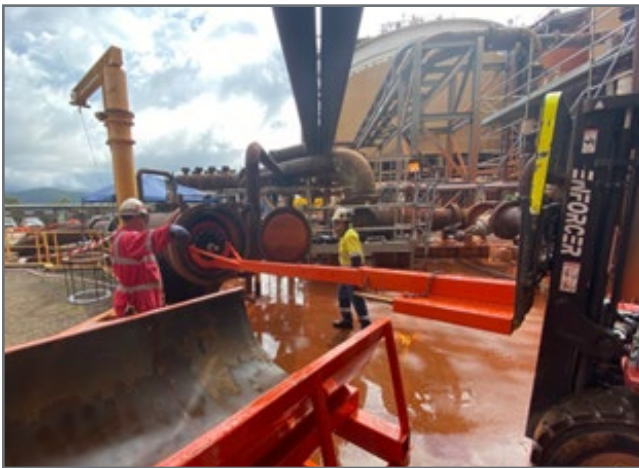
Figure 2: Launcher location during launch of gauging bidi
