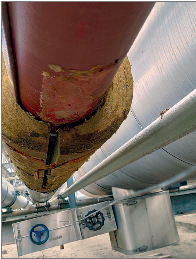
Figure 2: Corrosion was detected on the exact points that the CUI-CONTROL system pointed out.
