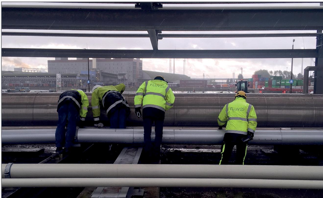
Figure 1: The Fluves engineers installing the sensing system on the MDI pipeline at BASF.
