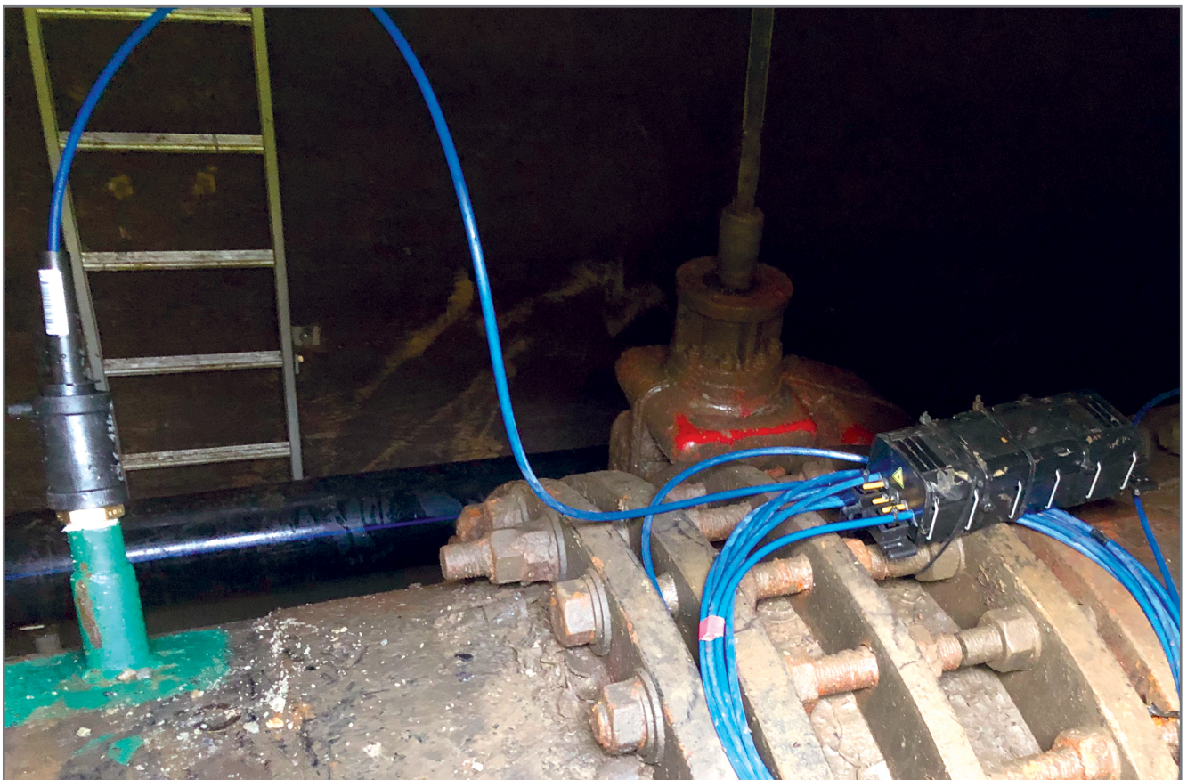
Figure 4 Fiber optic cable entering and exiting the pipeline to bypass a shut-off valve.
