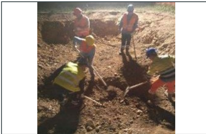
Figure 5: The manual digging operation, a typical preparatory activity anticipating the illegal tapping. This kind of events are detectable by the TPI system by exploiting the high sensitivity of the e-vpms® vibro-acoustic sensors.
