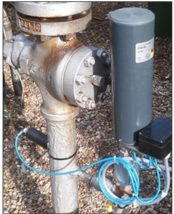
Figure 3: The e-vpms® sensor block mounted on an existing derivation.
