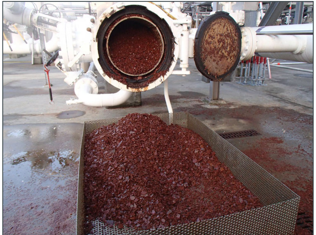
Figure 8: Picture Showing Receiver of the 14" Mining Water Pipeline
