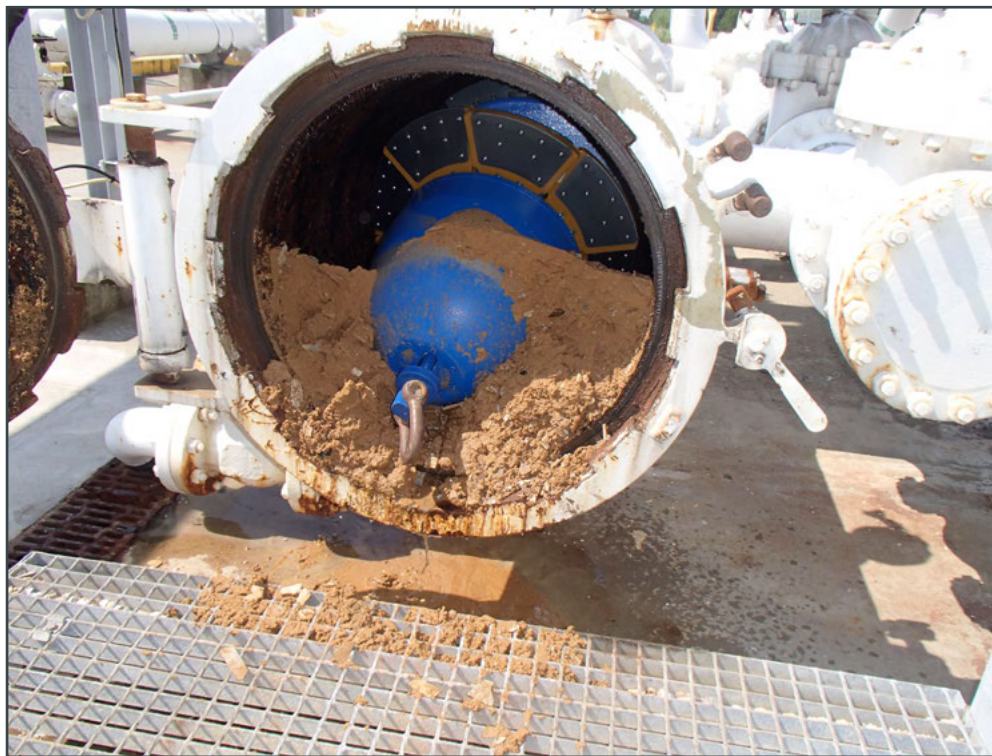
Figure 5: Picture Showing Retrieval of a 24" MCT Flushing Forward Powdered Scale
