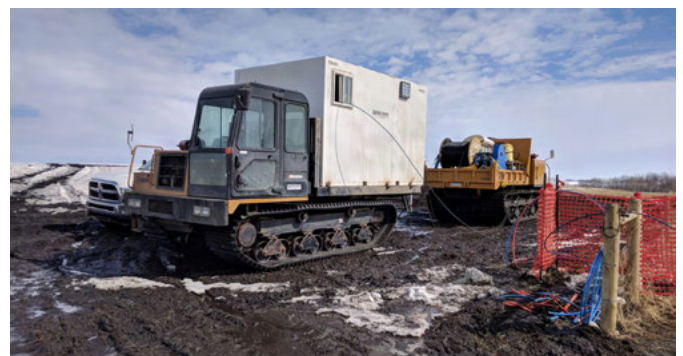
Figure 2 - Fiber injection at into buried conduit at a hand-hole site
