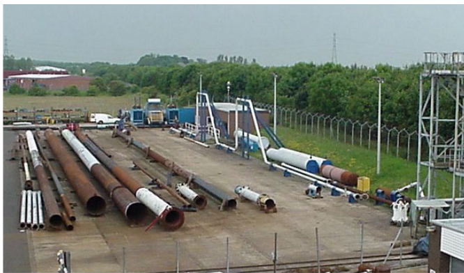
Figure F3.1 Pull through pipe spools with machined defects
