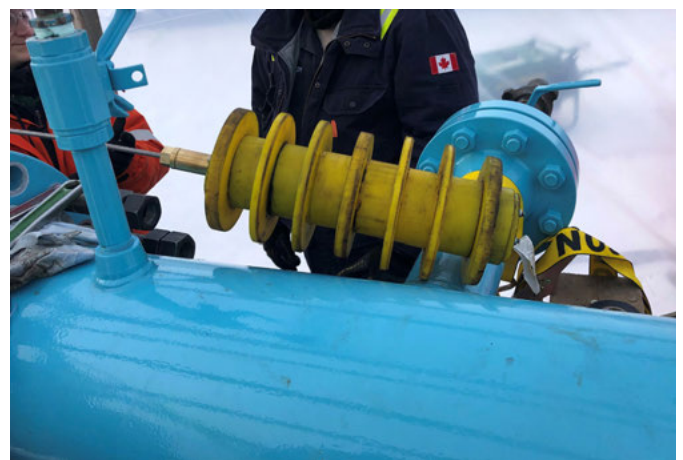
Figure 9 - Fiber optic cable attached to tow pig for internal deployment
