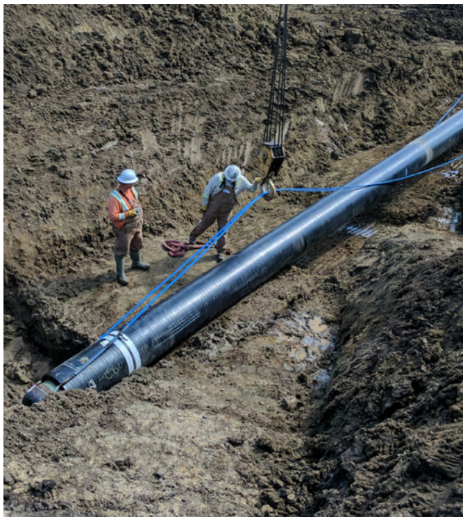
Figure 4 - HDD pull
