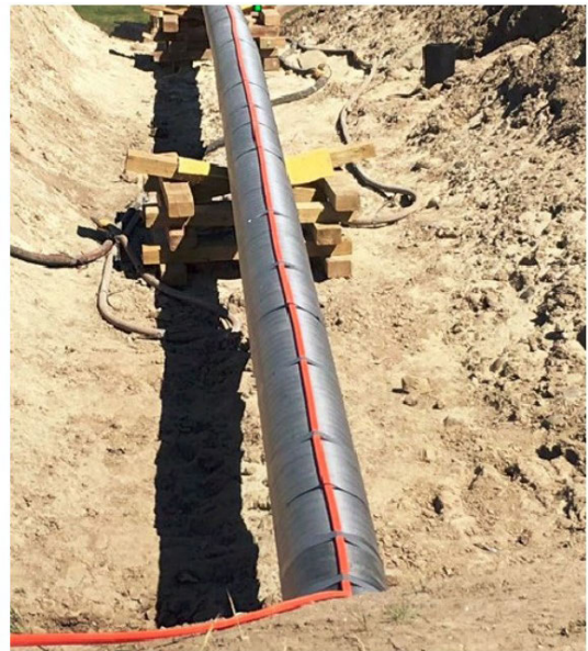
Figure 1 - On the pipe fiber installation
